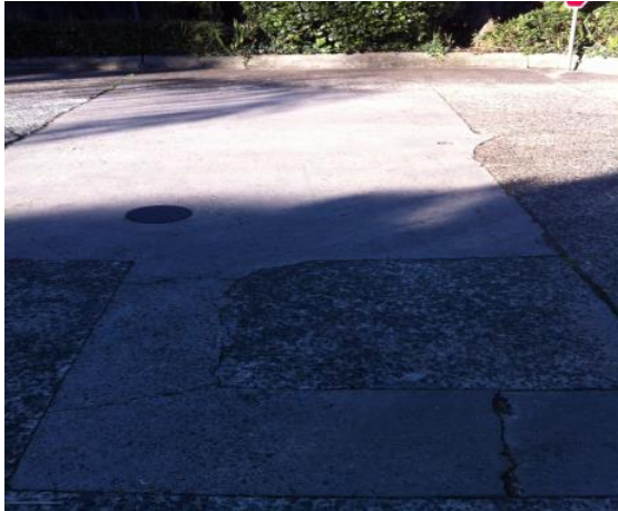
Photo 5.5.4 – Evidence of a decommissioned UST pit
