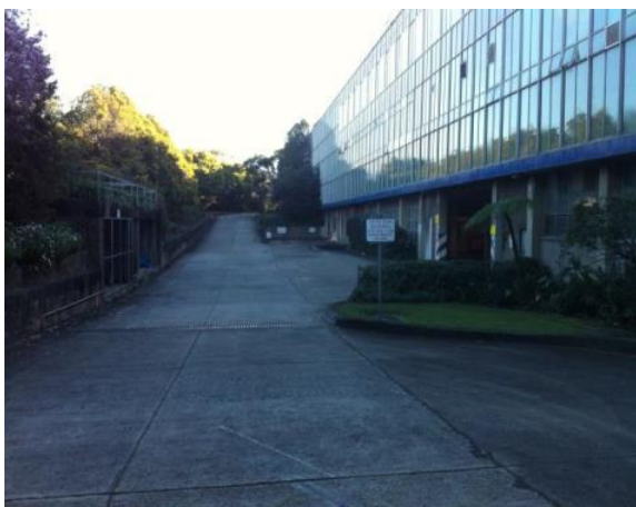
Photo 5.1.2 – Concrete driveway and the southern face of the current site building (looking west)
