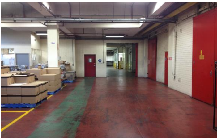
Photo 5.1.7 – View of the packaging material warehouse
