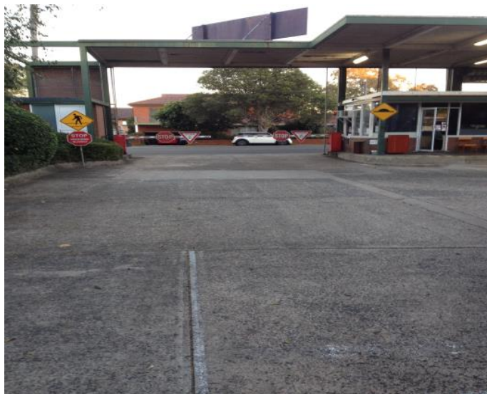
Photo 5.1.10 – View of the site's security shed – exit point
