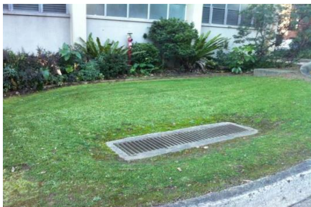
Photo 5.2.2 – Stormwater pit
